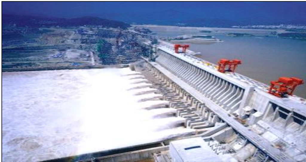
Fig. 3. Shows the Three Gorges Dam [59]
