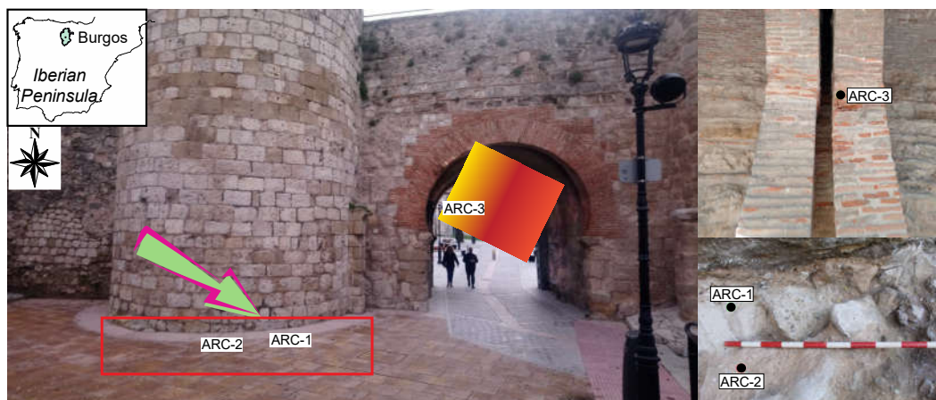
Figure 1. Sample location at the Arch of San Martin (Burgos, Spain). Arrows indicate sampling sites. Currently the ARC-1 and ARC-2 sampling site is covered.
