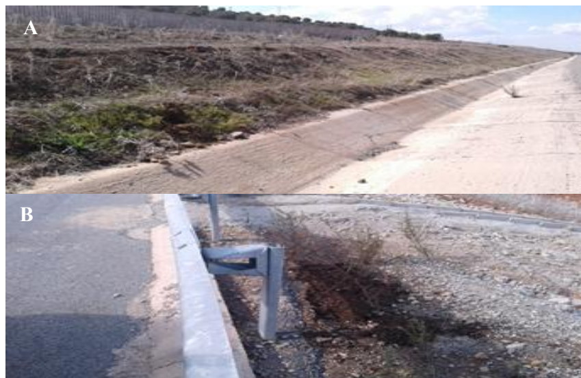
Fig. 1. Cut slope of Tahla (A), filled slope of Oued Amlil (B)
